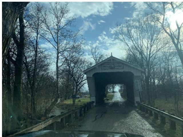
FIGURE 1-5 WARNCKE BRIDGE OVER SWAMP CREEK IN PREBLE COUNTY
